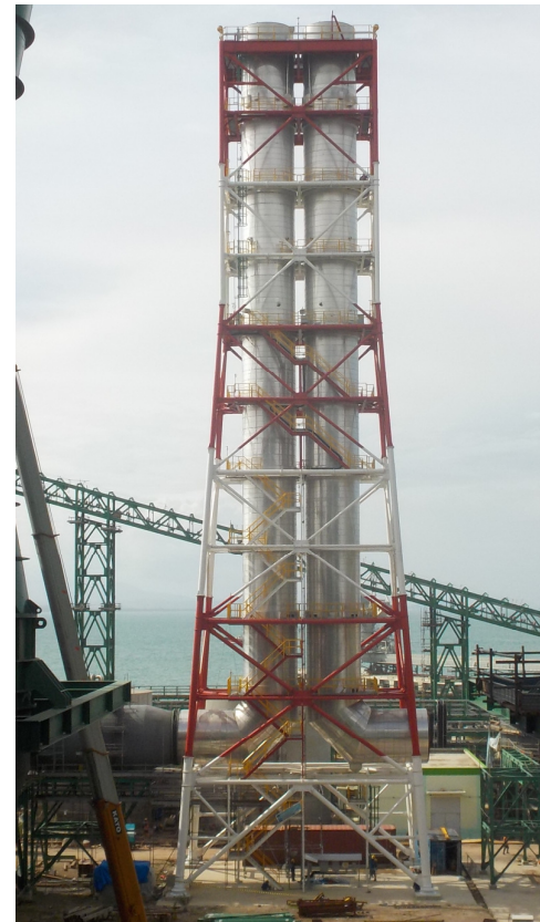
Completed Steel Frame Stack
