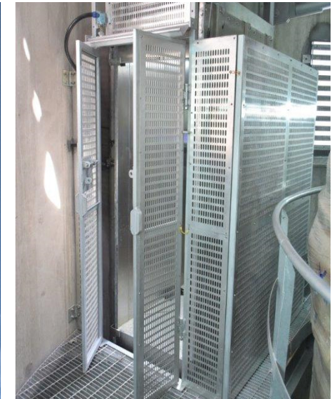
Supply & Installation of Rack and Pinion Hoist
