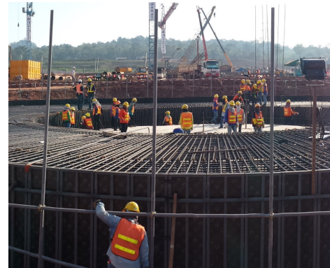
Pilecap Construction
