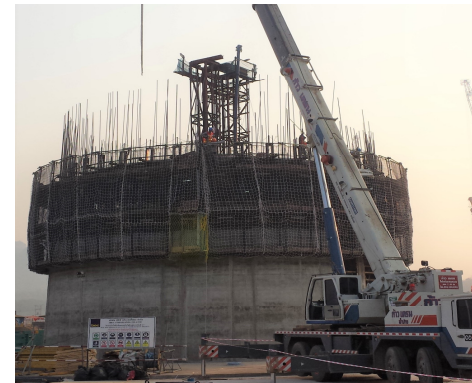
Concrete Windshield Slip-Forming in progress
