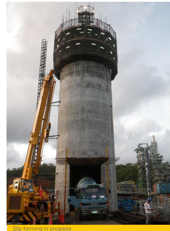
Slip forming in progress
