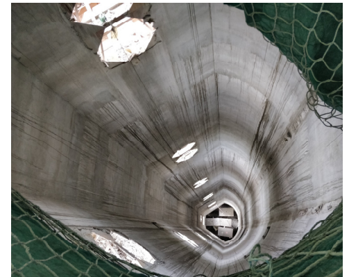
Internal of Tower Shaft
