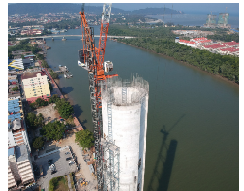
After Dismantle of Slip-form Equipment
