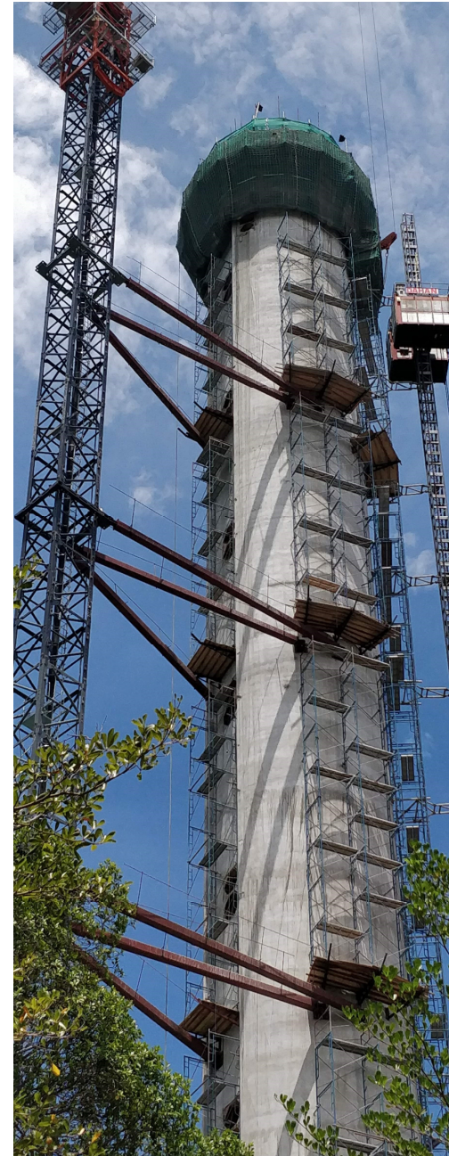
Tower Shaft Construction (Slip-forming)
