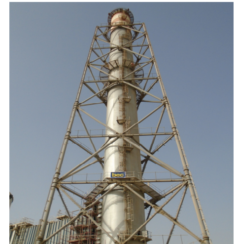
Inspection of Steel Stack
