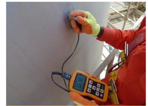
Ultrasonic Thickness Gauge Inspection
