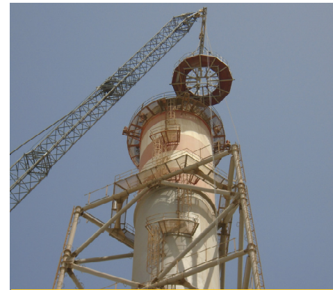
Lifting of internal access platform
