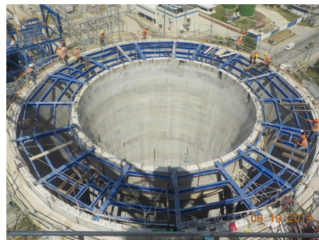
Roof Beams Installation
