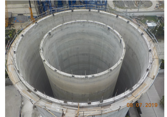
Dual Walls Silo
