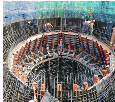
Construction of Internal Silo Cone
