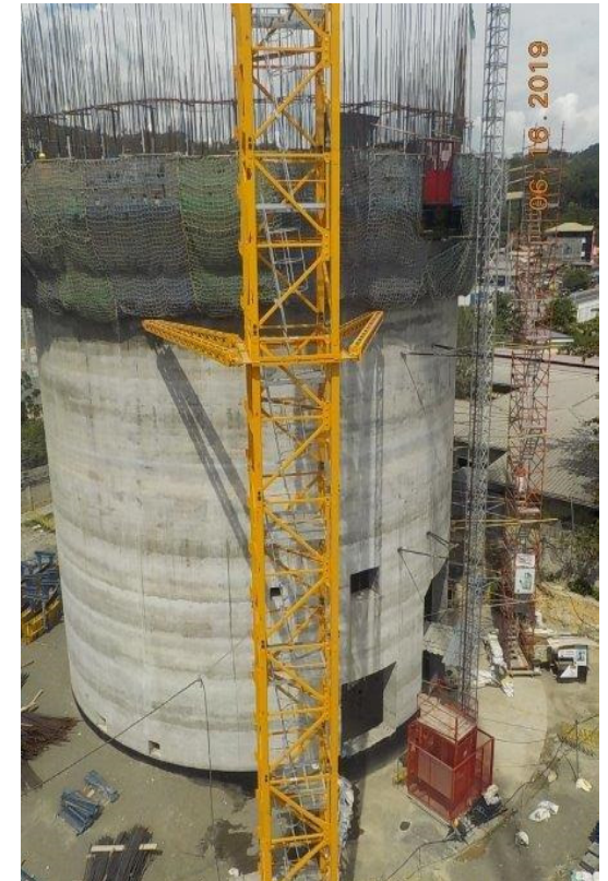
Slip-forming of silo wall
