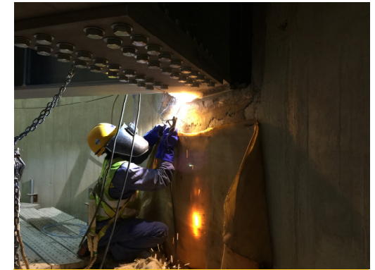
Installation of Floor Beam
