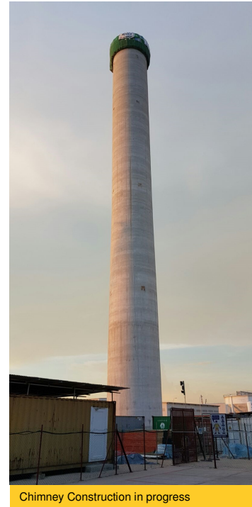
Chimney Construction in progress
