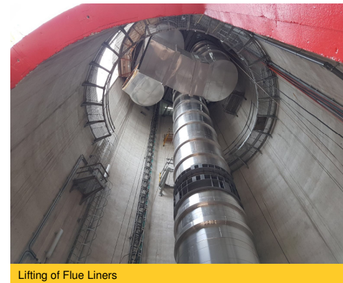
Lifting of Flue Liners
