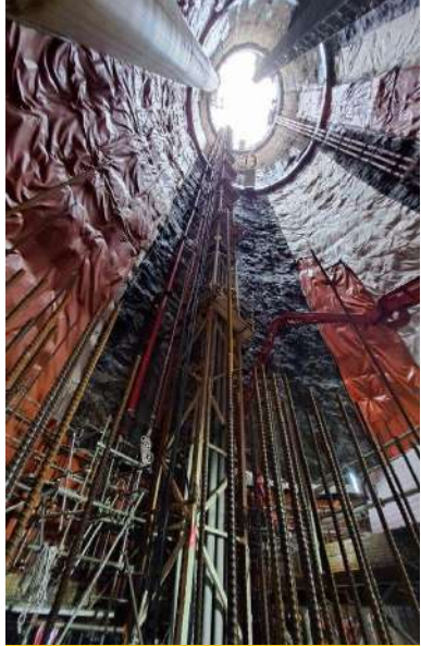
View looking up from the slipform rig
