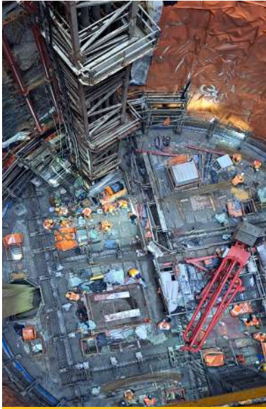
Plan view of the slipform rig
