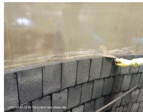
Borosilicate blocks installation
