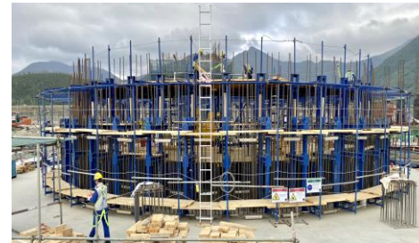
Slipform erection
