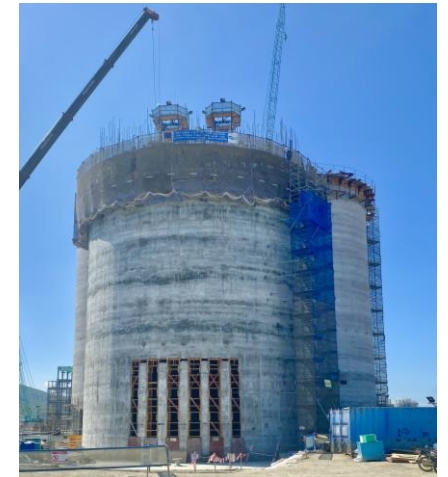
Slip-forming of silo wall
