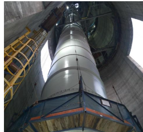
Lifting of flue liners
