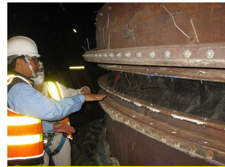
Removal of external insulation and installation of new expansion joint
