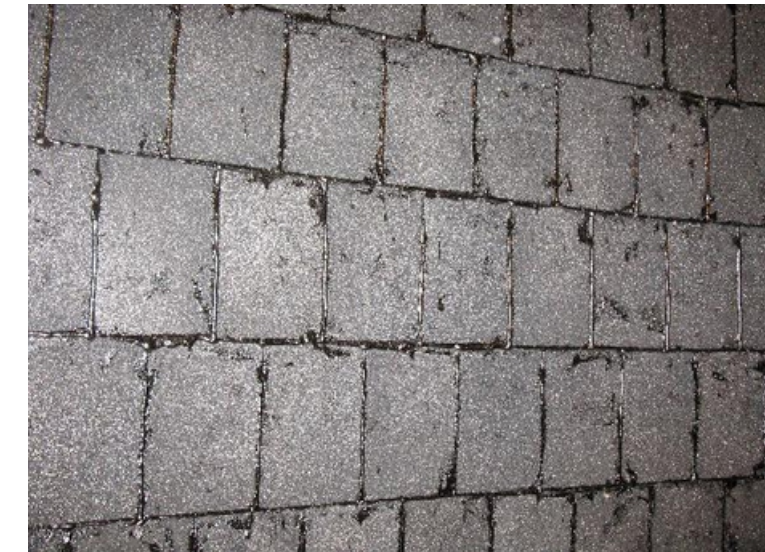
Installed borosilicate blocks
