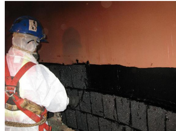
Laying of borosilicate blocks
