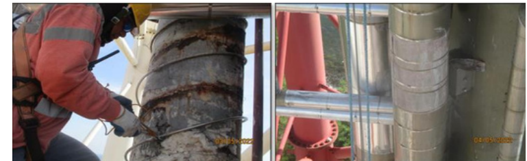
Repairing of leaking tracing line and cladding restoration
