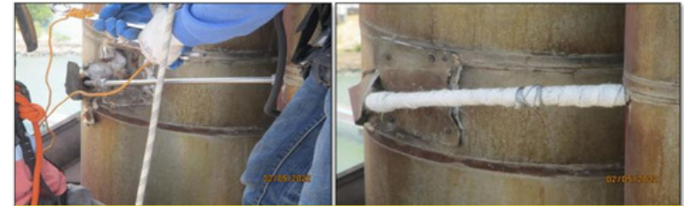
Restore damage insulation and cladding.
