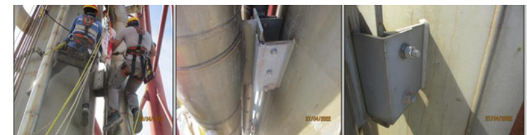
Support restoration and replacing missing bolts.
