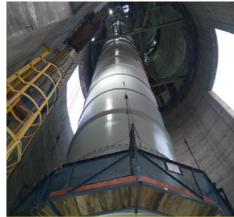
Lifting of flue liners
