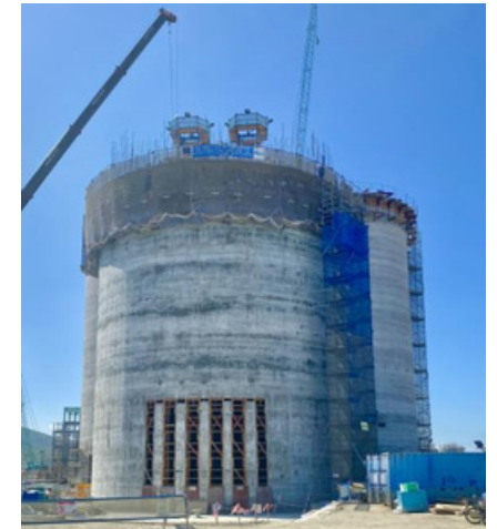
Slip-forming of silo wall
