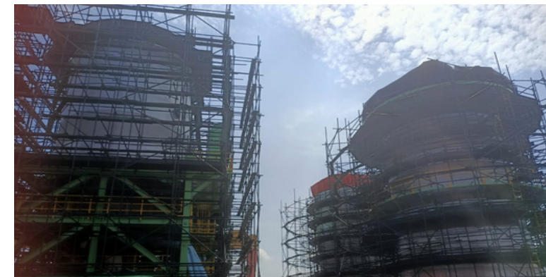
Thermal oxidizer section 1, section 2, and section 3, ready to lift and connect
