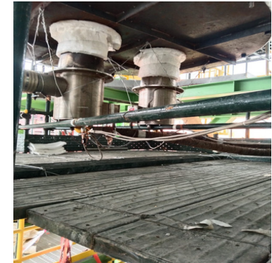
Refractory curing/dry out works to section 1
