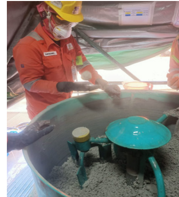
Testing and mixing of refractory material on site
