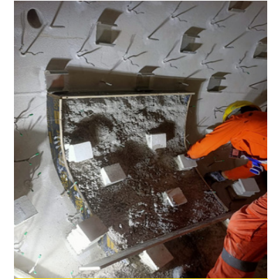
Installation of refractory material to section 1
