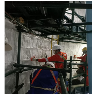
Installation of ceramic fiber module to section 2 and section 3
