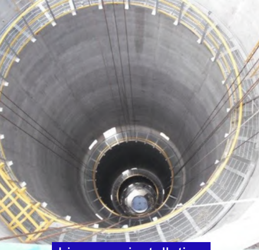
Liner can installation
