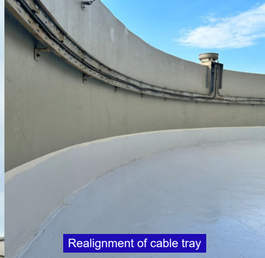
Concrete restoration to windshield
