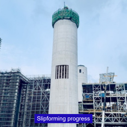
Sequential slipform construction of chimneys
