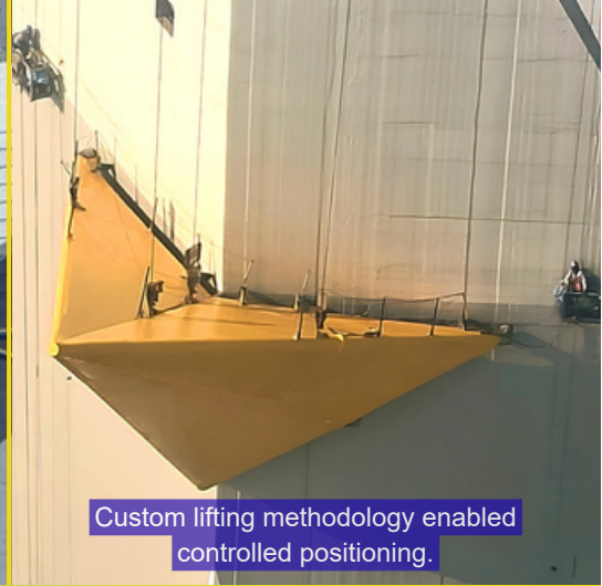
Pre-installed platforms and access points enabled safe fixation at elevation.
